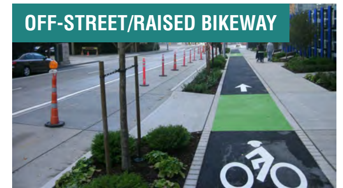
Off-Street/Raised Bikeway: Raised bikeways are vertically separated from vehicles and have markers, vertical separation, or barriers that separate them from the pedestrian areas.
