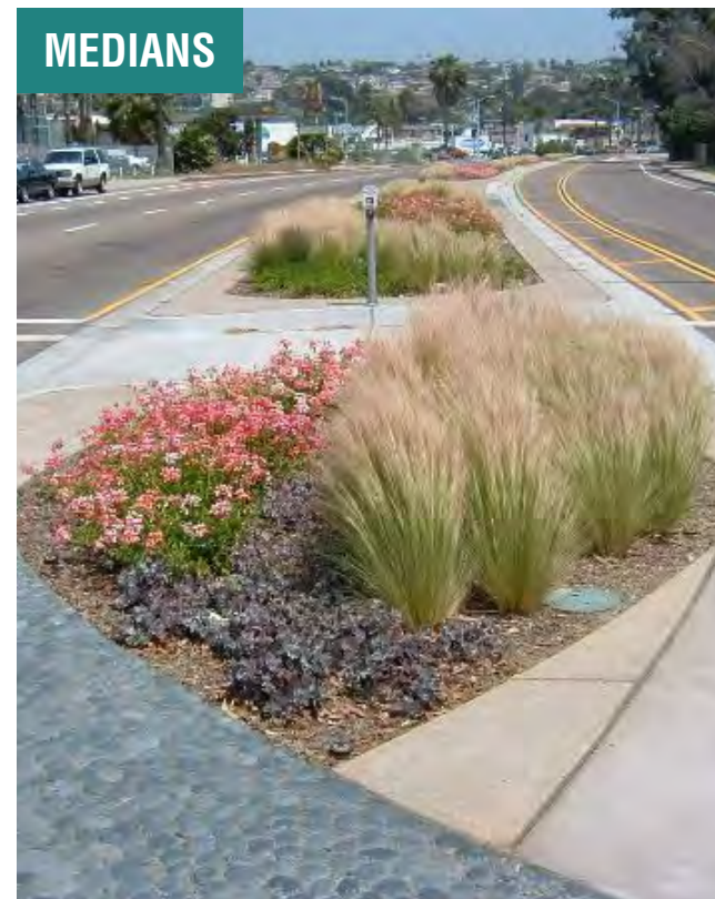
Medians: Medians are designed to separate opposing lanes of traffic and can come in many different forms. Common median types include raised, painted, and landscaped. The type of median is determined through engineering and cost-benefit analyses.
