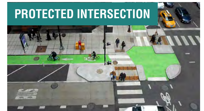
Protected Intersection: Protected intersections extend the physical separation between cars and people and provide dedicated bicycle signal time to reduce conflict and increase safety.
