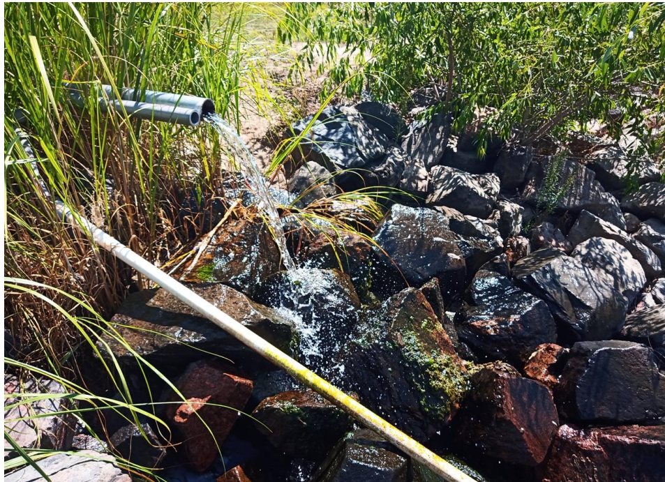
PICTURE 9. KETRING WELL DISCHARGE TO KETRING LAKE
