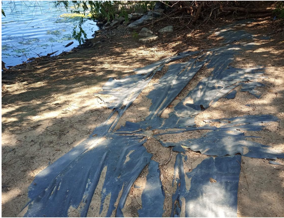
PICTURE 4. KETRING LAKE PVC LINER
