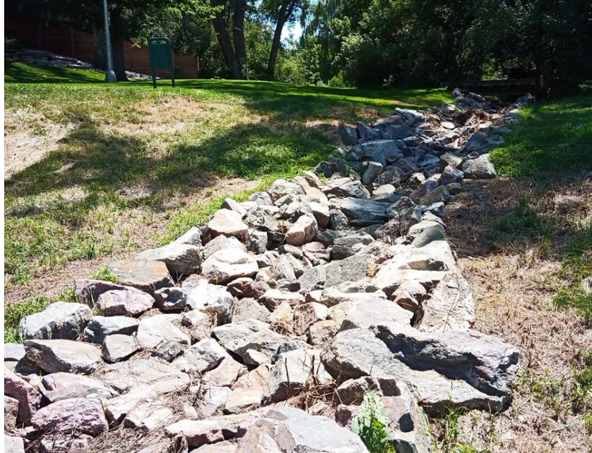
PICTURE 6. INFLOW CHANNEL TO RIDGEVIEW POND
