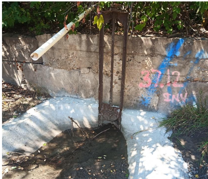
PICTURE 2. CITY DITCH HEADGATE ON SLAUGHTERHOUSE GULCH
