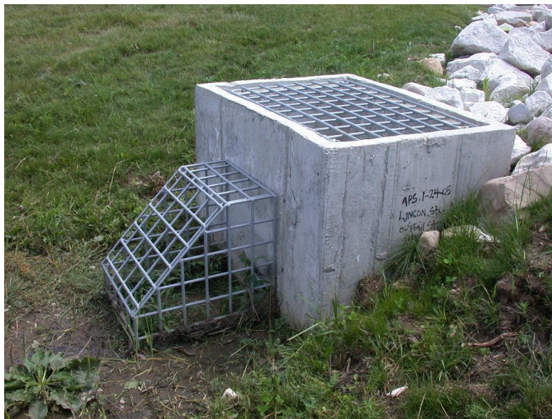
PICTURE 16. EXAMPLE RETENTION POND OUTLET
